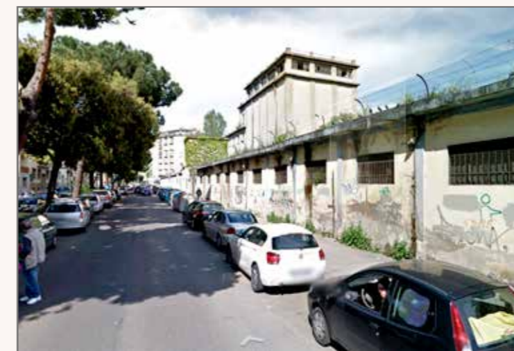
2) Side view of Via Mariti, where the complex is now enclosed by a boundary wall
