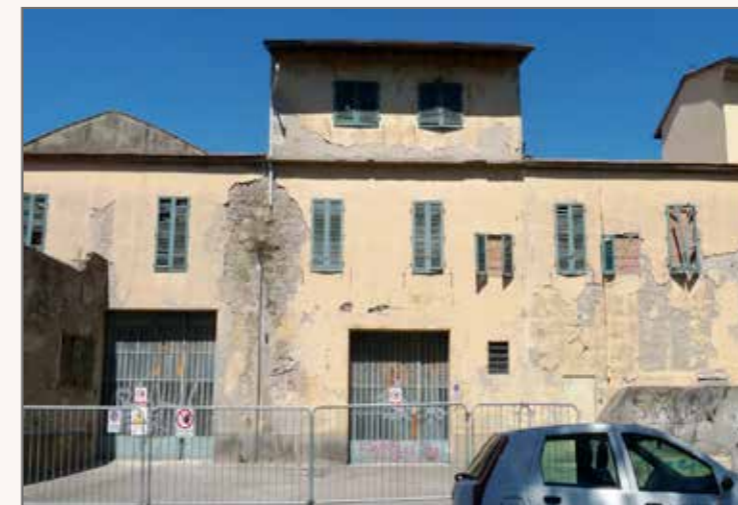
2) View of the side that faces Mugnone, now in a state of deterioration
