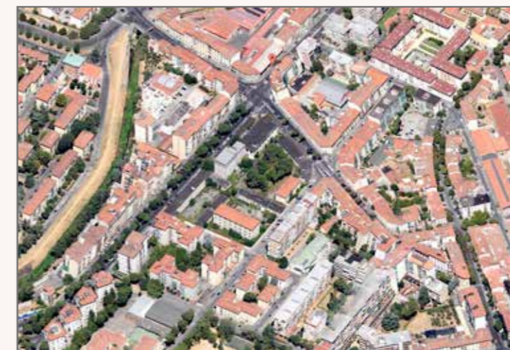
1) Overall view of the complex, which occupies an entire city block (recognisable by the dark roofs)
