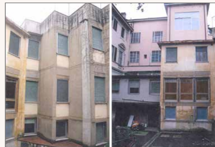
2) Views of the most recent additions, to demolish and rebuild from scratch
