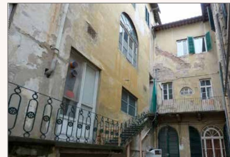
1 View of one of the inner courtyards, which overlook the parts in worse condition
