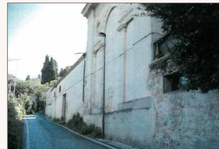
1) View on Via degli Incontri, with architectural elements of merit
