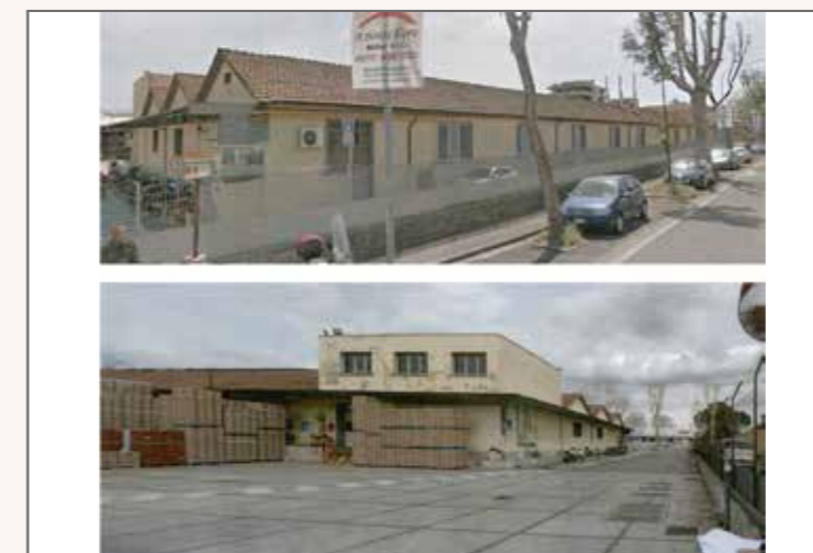
2) More images of existing buildings to be demolished
