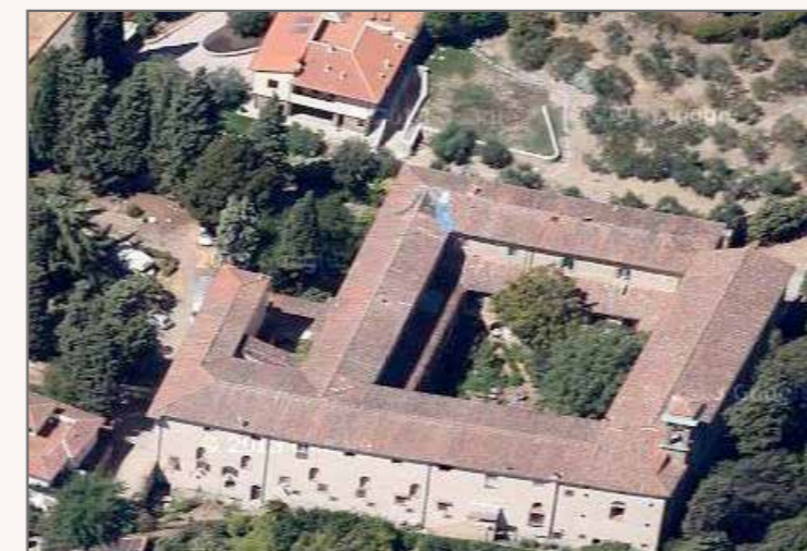
1) Overview of the complex immersed in the green of the hills south of Florence
