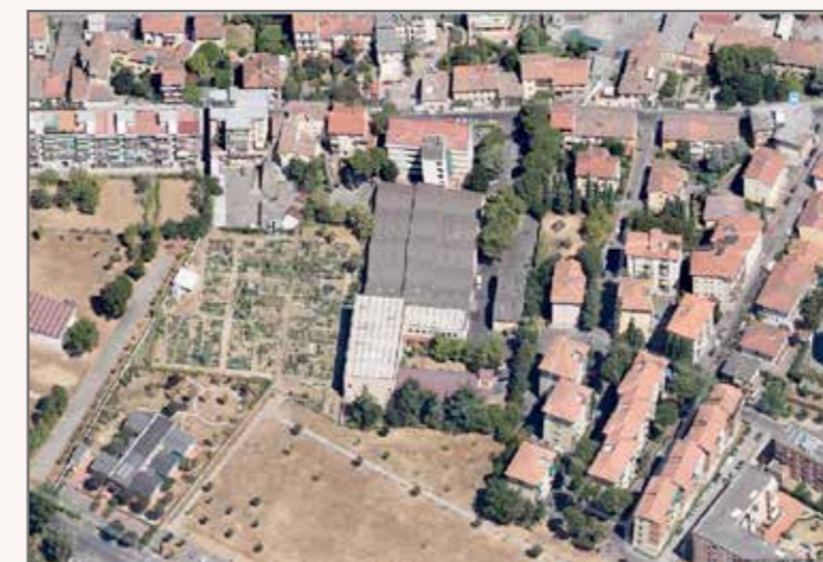
1) Top view of the industrial complex to be demolished; down, the adjacent public green area
