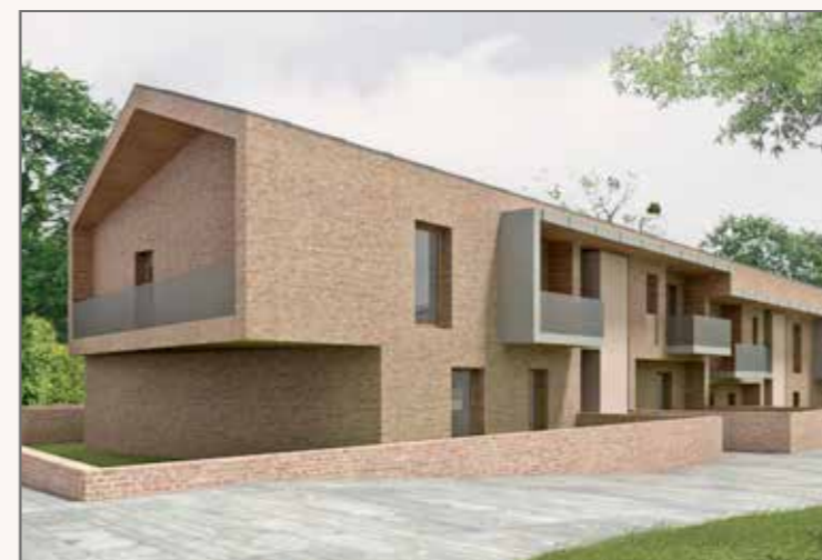
3) The architecture is geared towards energy sustainability and types that recall the rural construction, with extensive use of exposed brick
