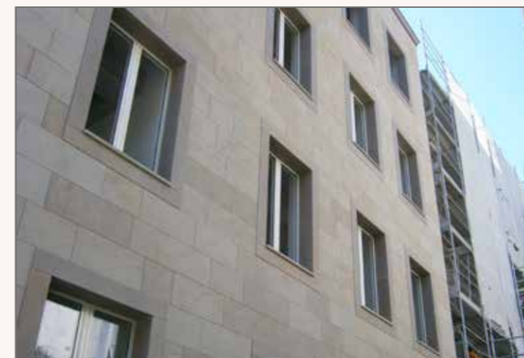
3) View of one already finished side, with lining in exposed stone
