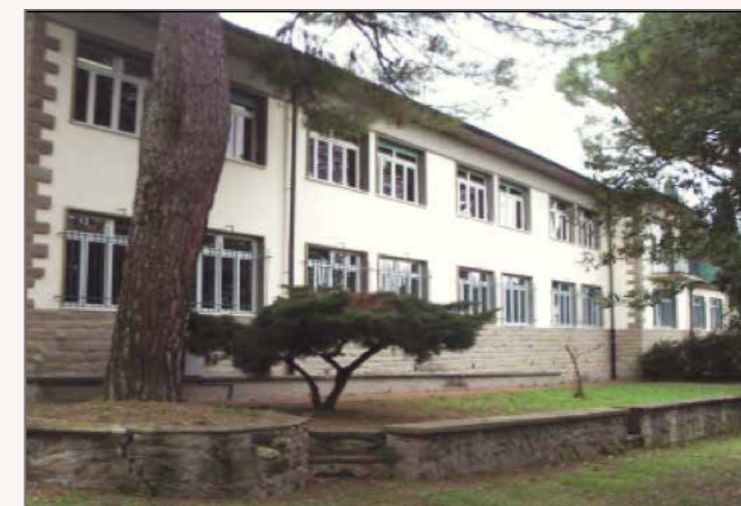
3) View of one of the buildings which demolition and reconstruction at equal volume has been permitted
