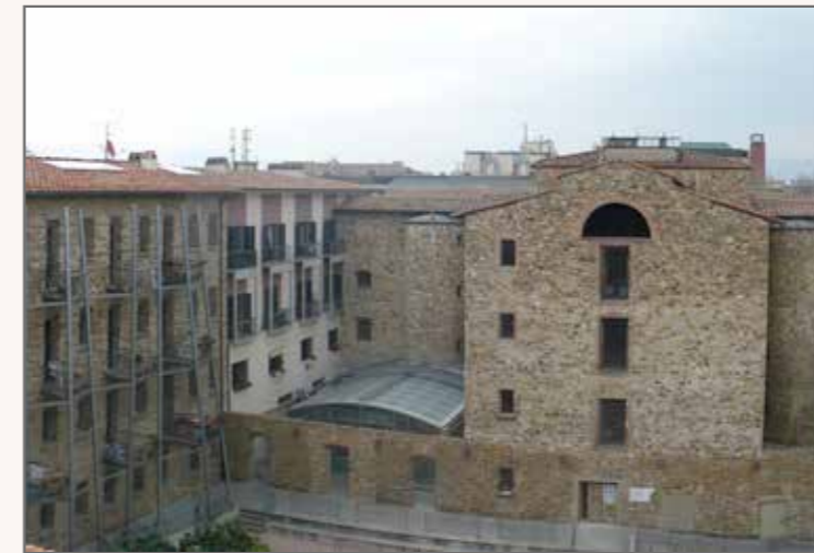
1) Overview of the main courtyard and the Convention Centre
