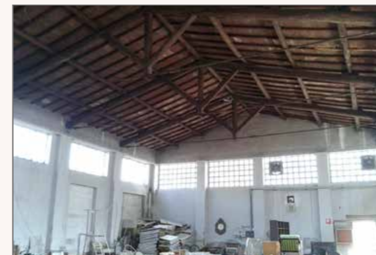
3) Interior view of one of the abandoned buildings, with wooden cover
