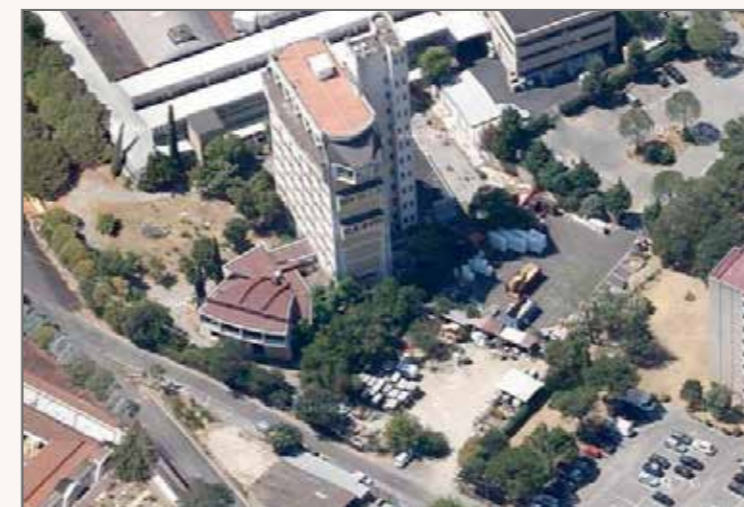
2) An overview of the main building (the tower) and the body of the hall with auditorium
