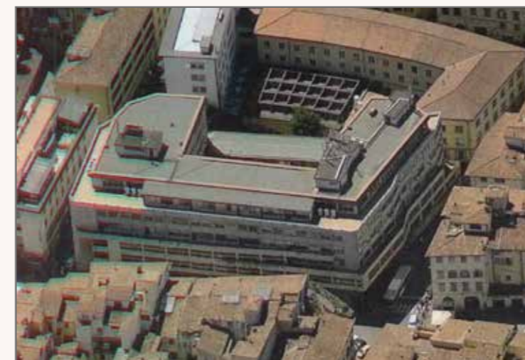
1) Overview of the complex, with a "U" shape around an internal courtyard
