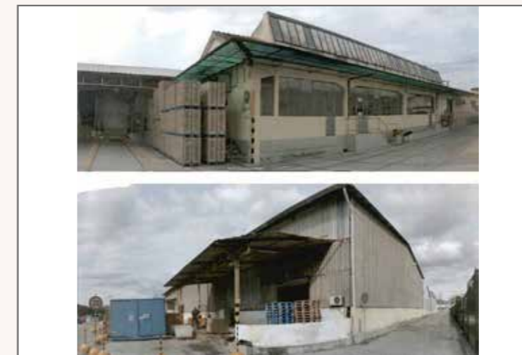
1) Views of the existing complex, in poor condition
