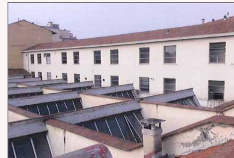
3) Seen from the inside, in the foreground the shed to be demolished and behind there is the two-storey building lined up on the access road
