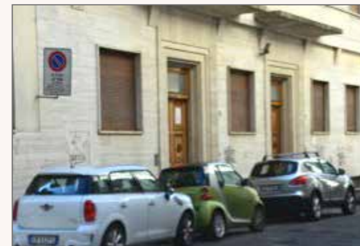
1) View of the main entrance of the building
