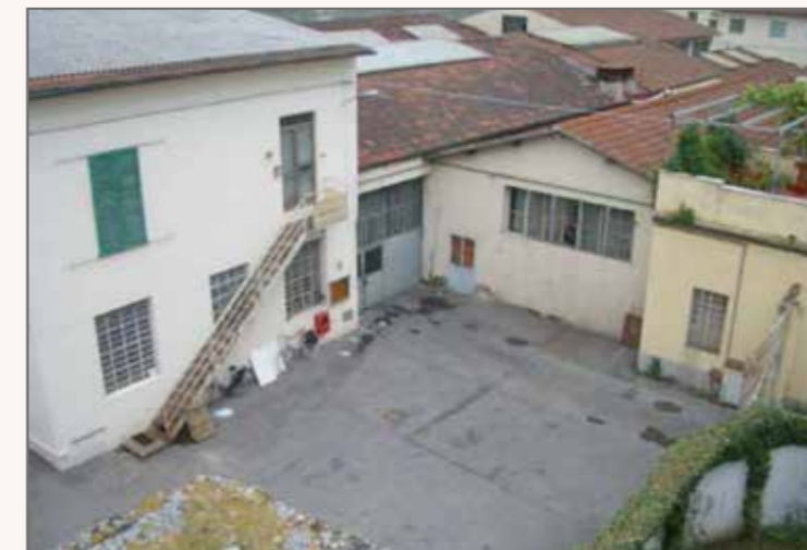
2) View of the central courtyard that links the various buildings
