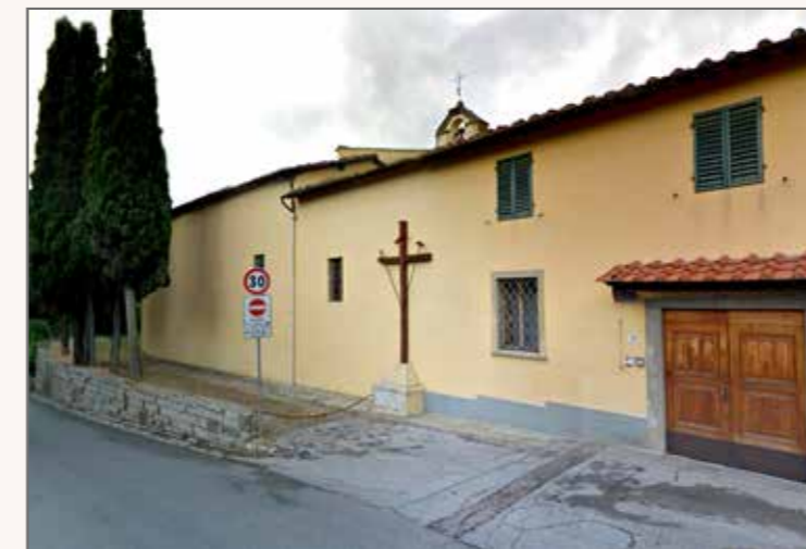
2) View of the entrance on Via dei Massoni
