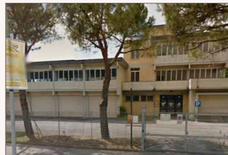
3) View of the main facade of the complex, which is still in good state of repair
