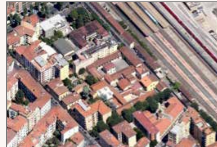
1) Overall view of the complex showing the proximity to the railway, and the compact surrounding urban fabric
