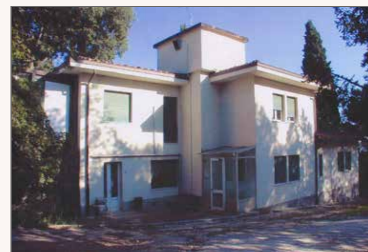
2) One of the recent buildings, for which the demolition and rebuilding with the same volume is scheduled
